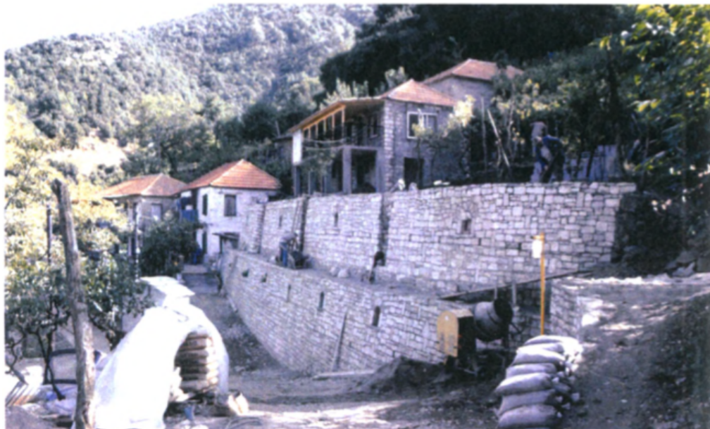
Construction of upper and lower wall for the landscaping above the square (Syllogos project), 1988-89.
